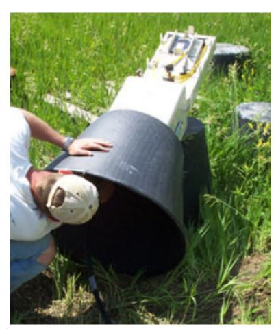
3.) With the cable pulled through the cone and pedestal, backfill with a 4" deep bed of pea gravel. Place the cone and pedestal in the excavation on the pea gravel bed. Place 4"-6" of pea gravel around the bottom of the cone. This will provide a barrier to rodents, and makes it easier to plumb the pedestal, which should be done at this point.
