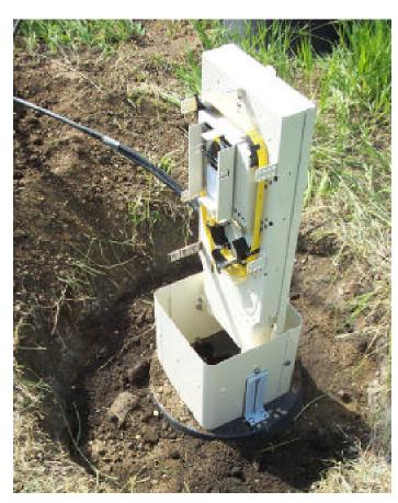
5.) When the splicing crew comes to the ped, they will pull the slack back out of the cone, and strip the loop cable to expose the buffer tubes. It is very important that the actual bend in the loop cable be in the portion of the cable where the jacket is removed.
