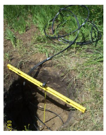
2.) Pass the grouped cable up through the opening of the BPS cone. It is important that the tightest part of the loop as it passes through the cone be within the length of cable that will later have the jacket removed.
